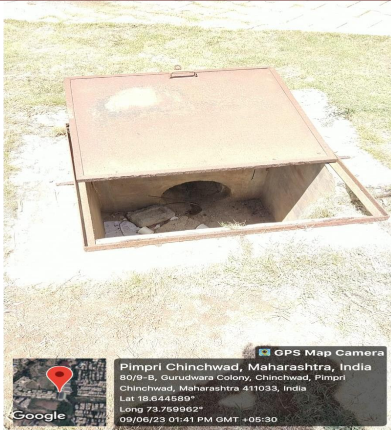
Pits for Rain Water Harvesting
