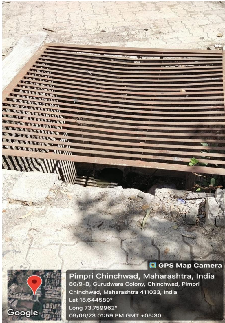
Primary stage of collection of sewage water
