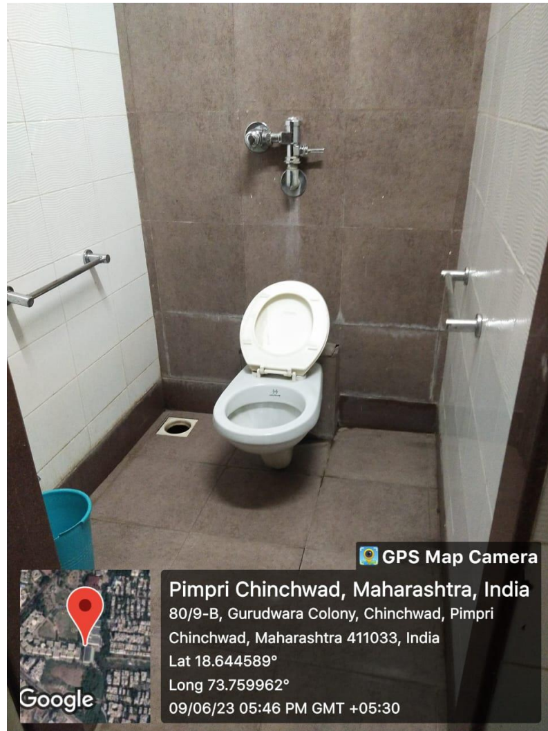
Provision for Disabled friendly washroom is provided
