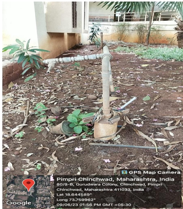
Borewell for digesting rain water
