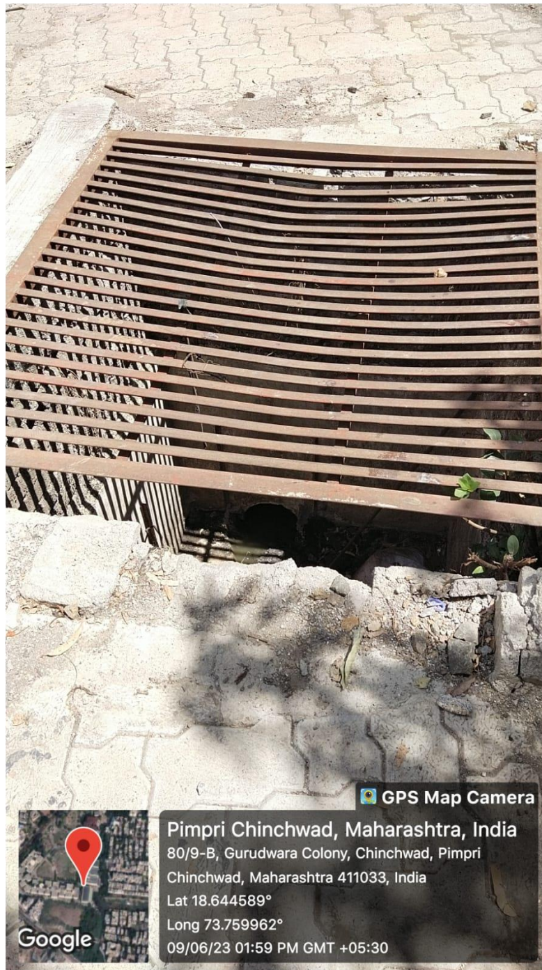
Primary stage of collection of sewage water
