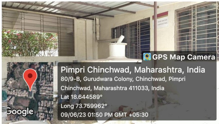
Rain Water Harvesting Plant
