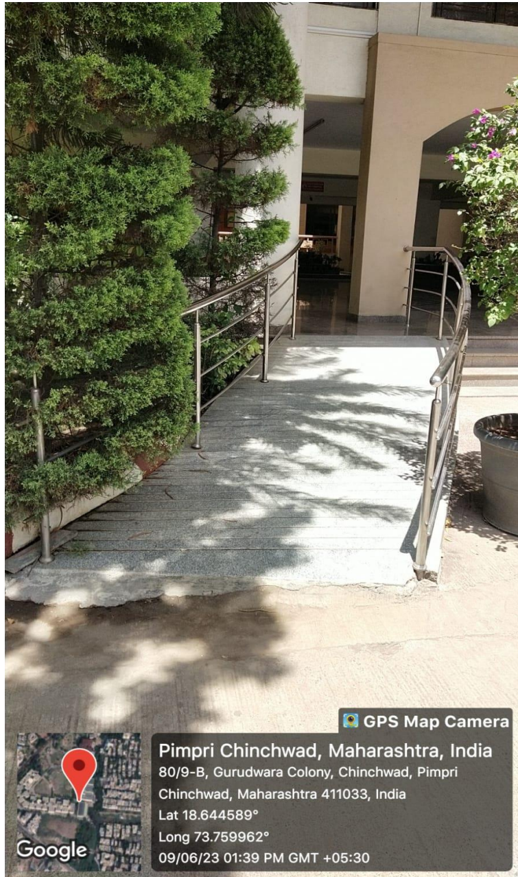
Ramp and rail constructed at the entrance for ease of access to disabled students, staff and visitors
