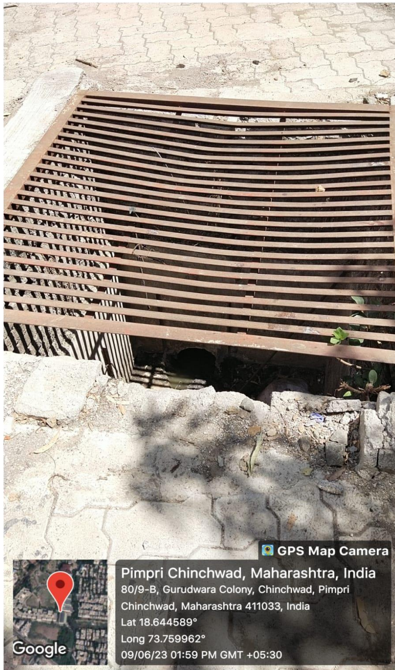
Primary stage of collection of sewage water
